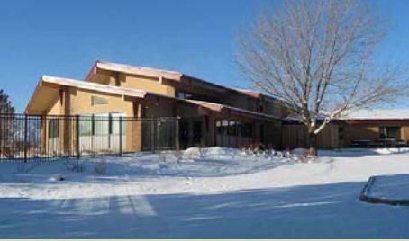
McCandless State Veterans Nursing Home (Boulder Associates, Inc.)
