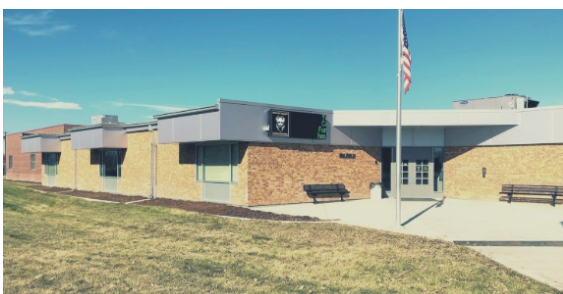
WELD RE-1 SOUTH VALLEY MIDDLE SCHOOL RENOVATION Location: Platteville Architect: Treanor HL
