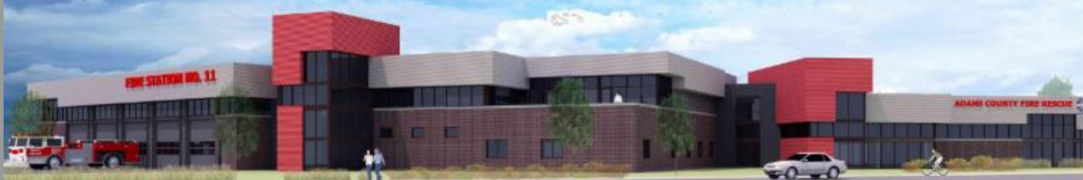
ADAMS COUNTY FIRE STATION NO. 11 - UNDER CONSTRUCTION
