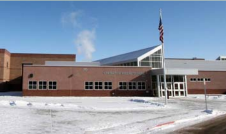
Creighton Middle School (CSNA Architects)
