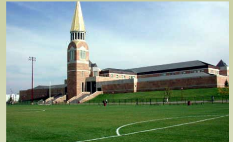
DU Athletic Complex and Art Annex (Tryba Architects)
