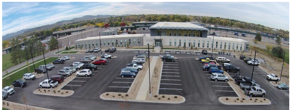
Loveland Service Center
