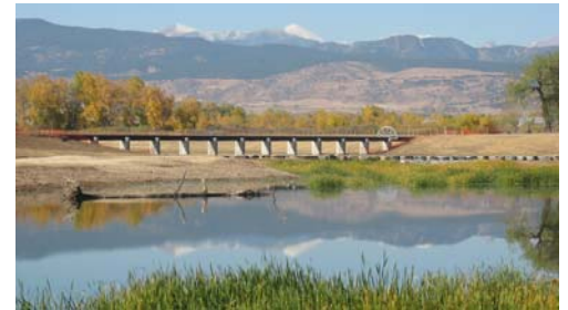
Lykins Gulch Stream Restoration (Ayres Associates)
