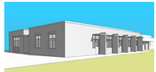
Ryan ES Renovation/Addition (RB+B Architects, Inc.)
