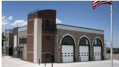
West Metro Fire Stations #4 & #8 (OZ Architecture)
