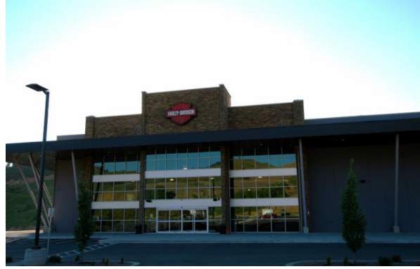
Avalanche Harley Davidson Core and Shell and TI - Gateway Village Location: Golden Architect: G3 Architecture
