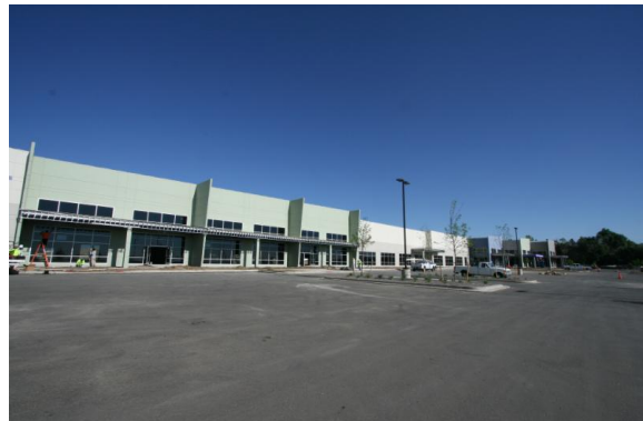
633 CTC Core, Shell, and Site Improvements (633 CTC Flex Warehouse) Location: Louisville Started: June 2016 Architect: MOA Architecture
